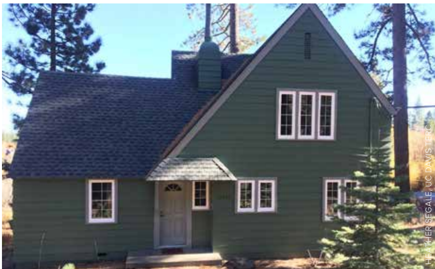
Malyj Manor (formerly the "Blue House") has provided lodging for graduate students and visiting researchers for decades and recently received several major upgrades by UC Davis Facilities
