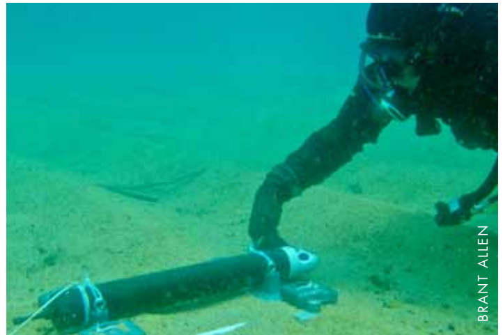
TERC research diver installs acoustic current meter to measure complex flows across the sill at the mouth of Emerald Bay
