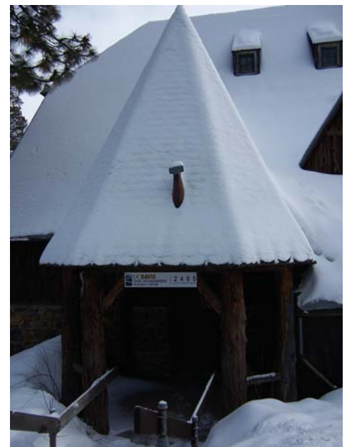
TERC staff ready for major renovation of historic hatchery site beginning July 2006.
